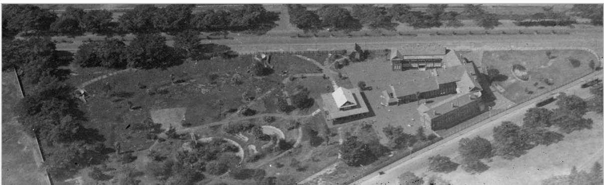
Aerial view of SGHS within the old Moore Park Zoological Gardens site between 1921 and 1926. Detail from Milton Kent aerial photograph, Mitchell Library of the State Library of New South Wales.
